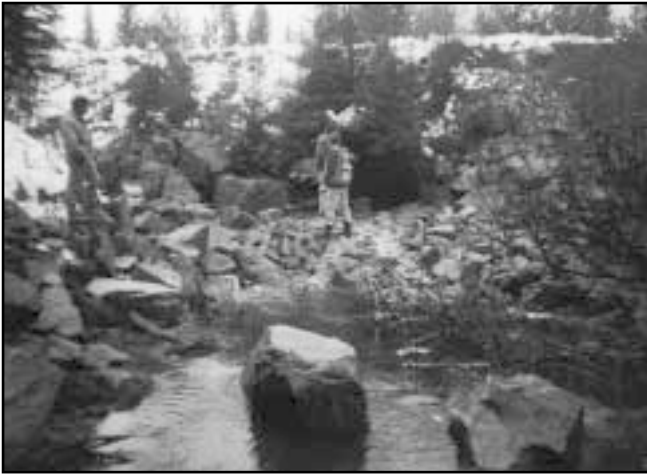
Figure 5. Rock riffle from culvert outlet that formerly had a 0.54 m drop.
