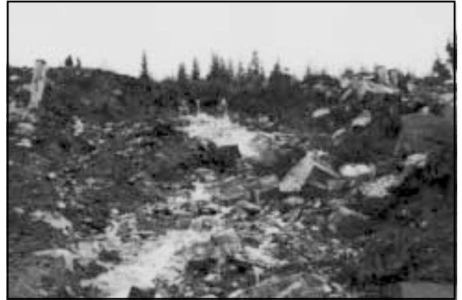
Figure 3. Photograph of the slide's initiation zone. Note the planar nature of failure surface, high cut tree stumps supporting road fill and abundance of water flowing over the headwall of the slide.
