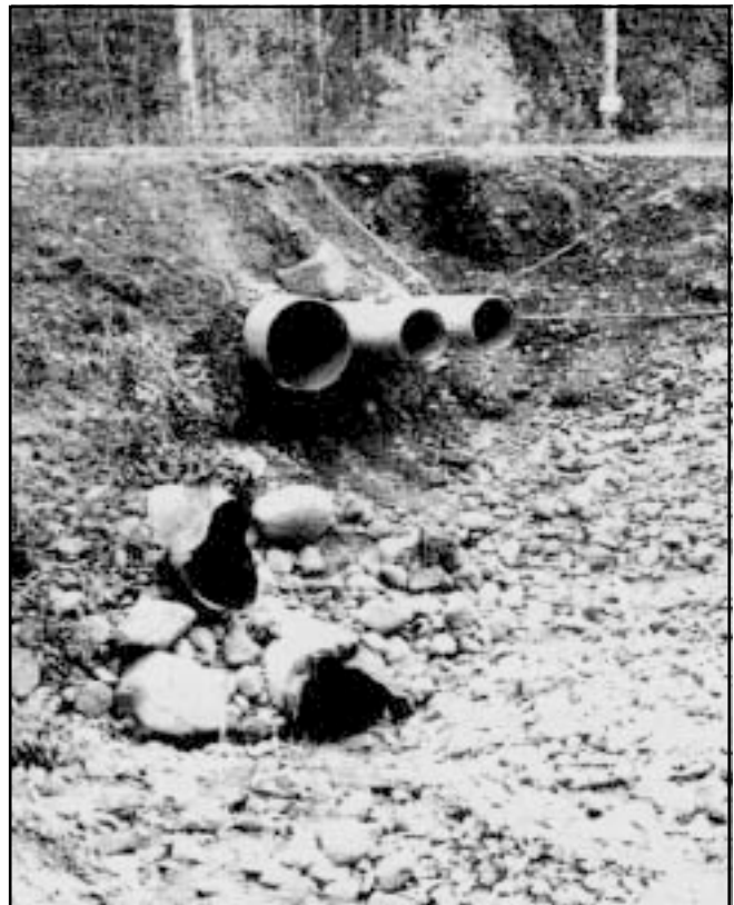
An example of fish barriers caused by road construction: Central and Northern Interior Fish Access by Michael Parker (see page 9A).
