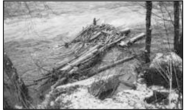
Figure 5. Debris groin at Coquitlam River in winter, 1999. The height of the groin should be just above floodplain height to prevent debris washout.
